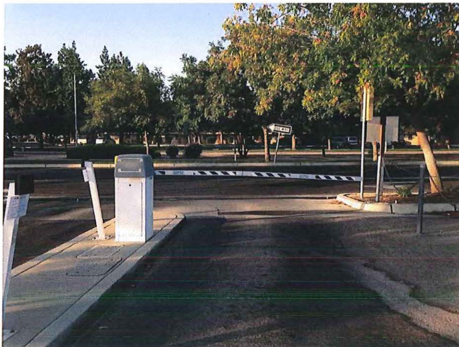
Employee Lot Exit Gate
